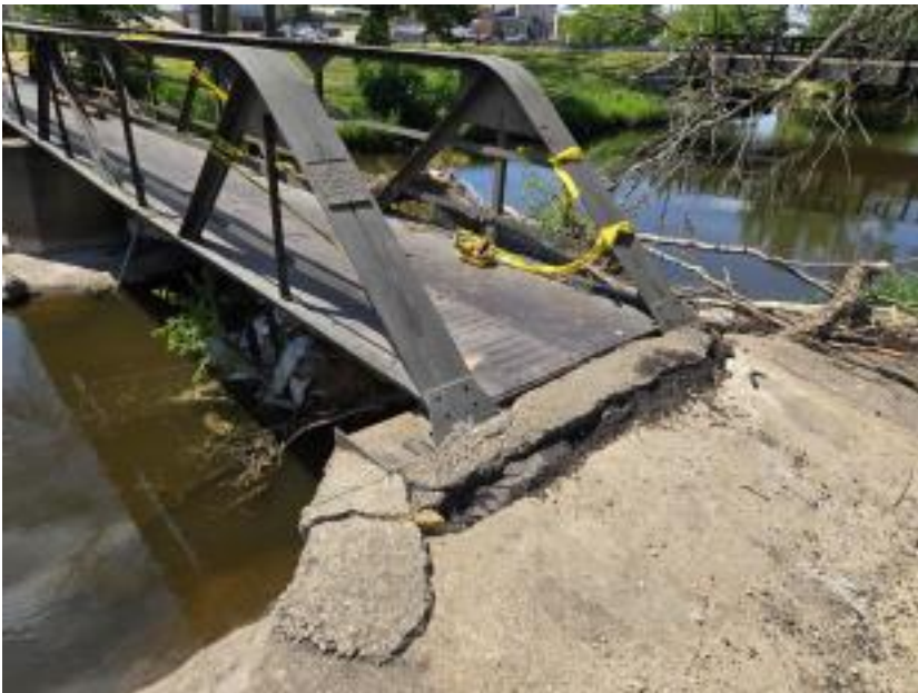
Northeast end of deck Meeting abutment
