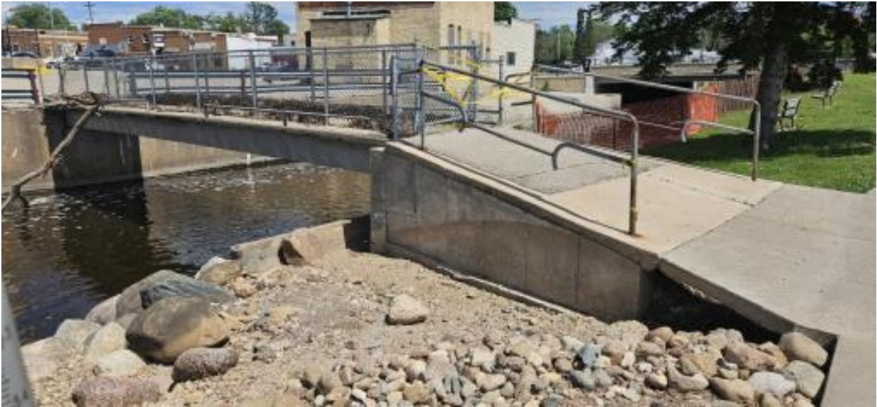
South side of Bridge looking NE
